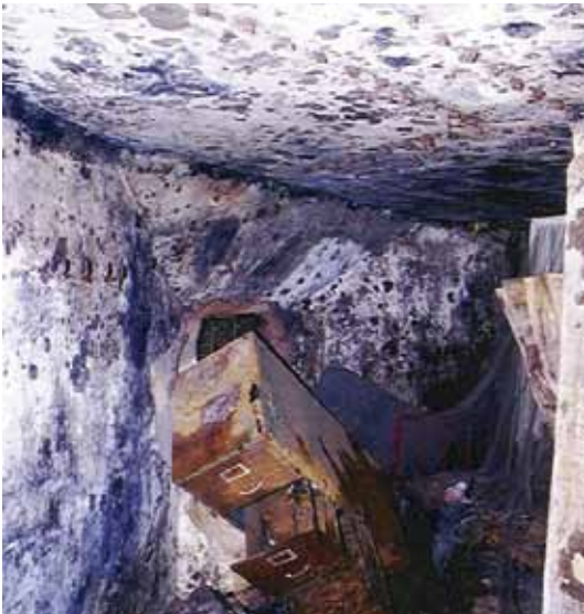
Figure 12: The right firing loop and part of the living space can be seen on the right side. Note the mark on the ceiling for the ventilation duct mounting and the hook on left side wall.
