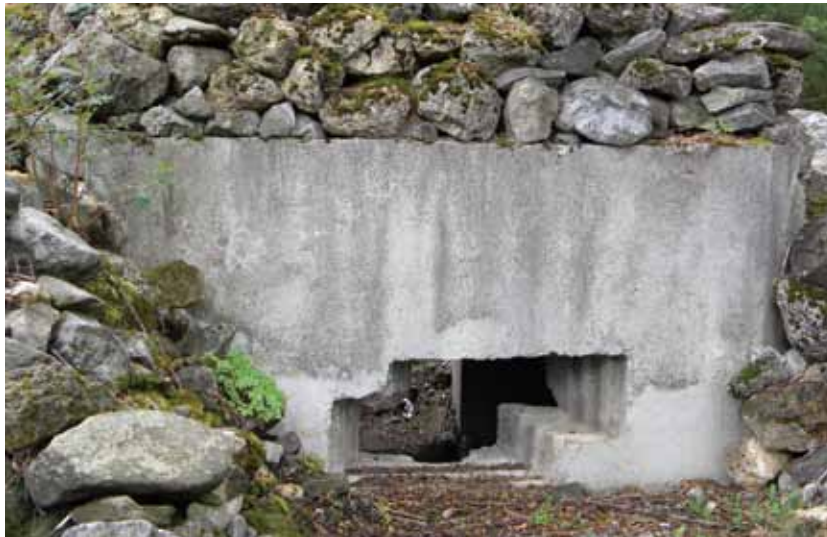
Figure 4: A French pillbox dating from 1939, probably for a 25mm anti-tank gun, at La Vachette close to the Italian border in the south east of the country. Associated with this work were shelters, infantry pillboxes and mine chambers forming a valley barrier and part of a network of defences along the border.
