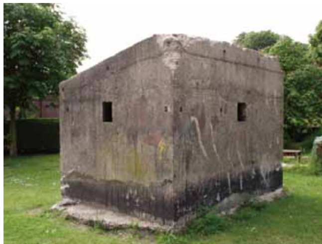
Figure 11: A British 1940 pillbox preserved at Whittington Barracks, Staffordshire. This unique design, to resemble a railway platelayer's hut (it would have received wooden cladding), was removed from its original position on the River Tame stop line.
