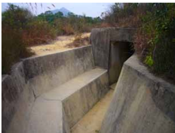
Figure 15: Trench near Strand Palace Hotel the kitchen of Shing Mun Redoubt Location E in Map 2. There are a number of similar open air trenches linking and in between the 'Underground' Tunnel System. These used for gun and mortar firing. This location is close to kitchen area and Charing Cross. [Editors' notes: T3, Figure 2, Lai, Ching, Davies and Wong (2011), this issue.]
