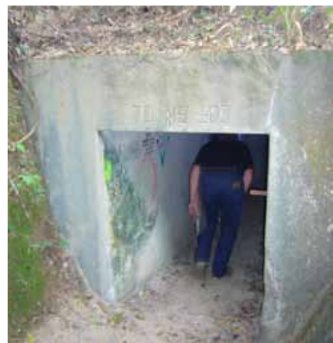
Figure 13a: Hay Market tunnel to PB403, Sing Mun Redoubt Location G in Map 2.
