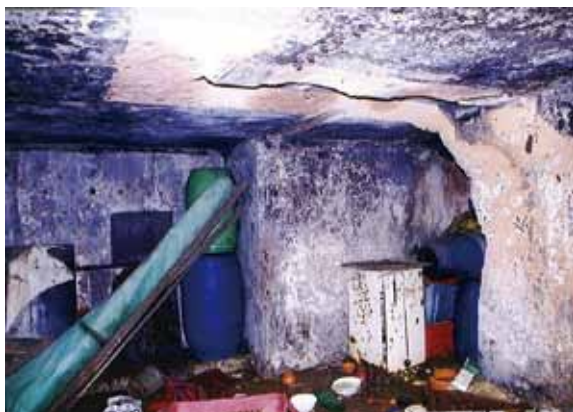
Figures 10a & 10b: The back room and entry. Note the demolished middle wall and the slot on the roof in front of the entry.
