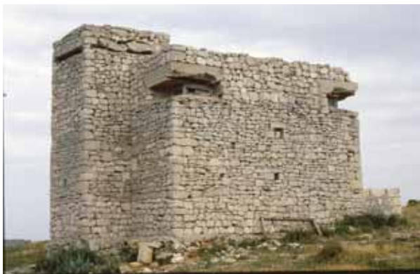
Figure 5: A British pillbox on Marfa Ridge, Malta, dating from 1935. It is carefully camouflaged with stone to resemble local buildings. The corner embrasures for machine guns are a characteristic of Maltese pillboxes. Note the observation position in the top of the ventilator.
