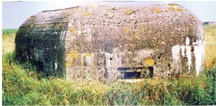
Figure 7: A reinforced concrete pillbox built by the British Expeditionary Force at Cysoing, northern France in 1940. It has three machine gun embrasures. (Courtesy: Dr Mike Osborne).
