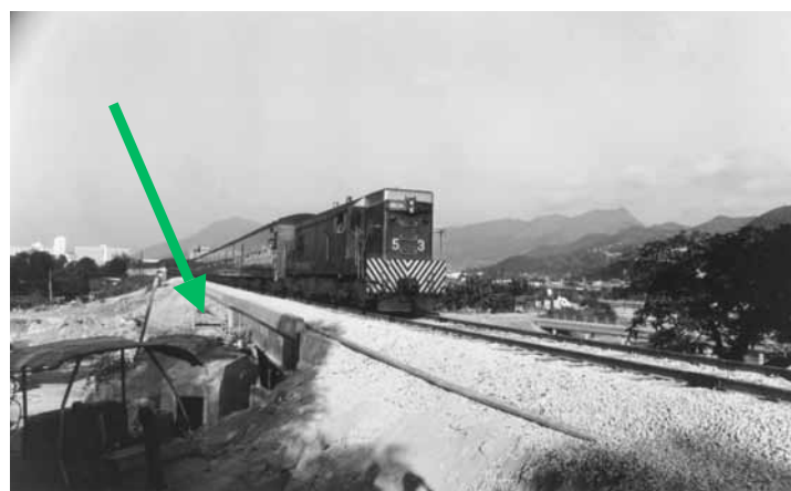
Figure 2: PB 304, Gin Drinker’s Line, Tai Wai Railway Bridge, 1976
