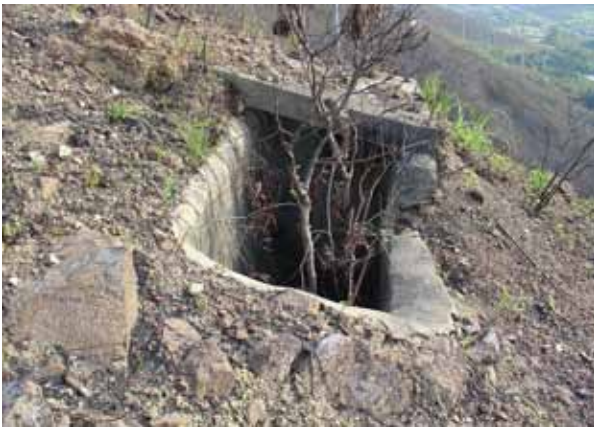
Figure 19: Concrete post, Pok Wai
